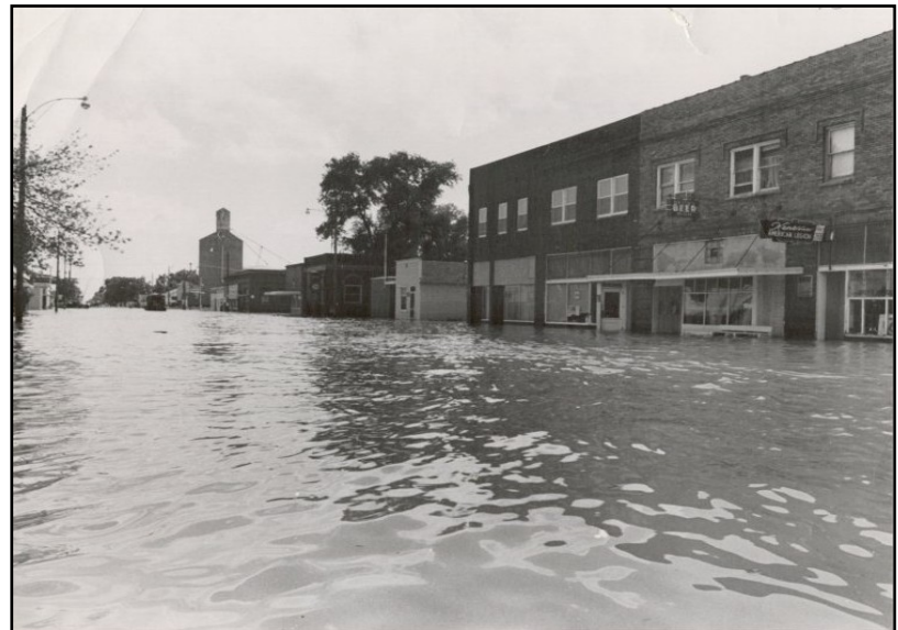
Downtown Kenesaw, 1967. Flash flood on 32-Mile Creek.
